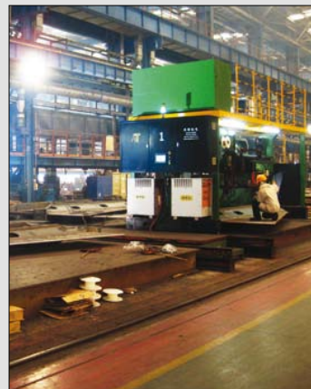
Multiple gantries effectively moving to different shape beams along the rails
