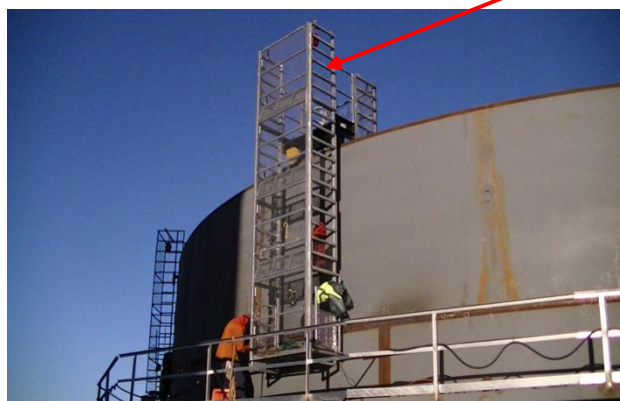
Additional cross members have been added from the top to the bottom of the frame and spaced to work as Ladder Rungs built into the Shell buggy frame so the operator can easily and safely climb between the levels.
